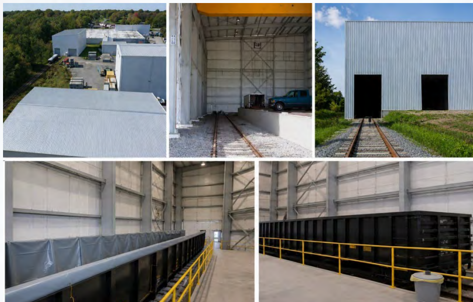
Containers staged for sort, segregation, and consolidation at the WCS Alaron Facility.
